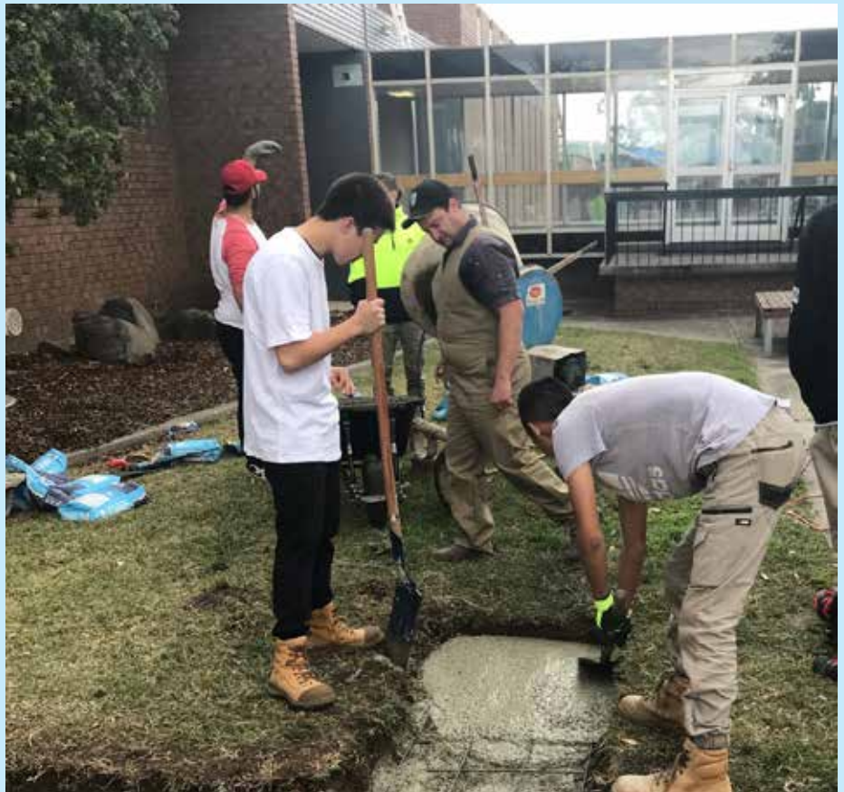
Preparing the ground and pouring the concrete for a bricked-in BBQ.
